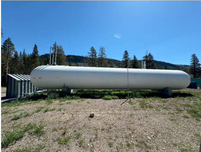
Figure 3.2: Existing Storage Tanks (looking east)
