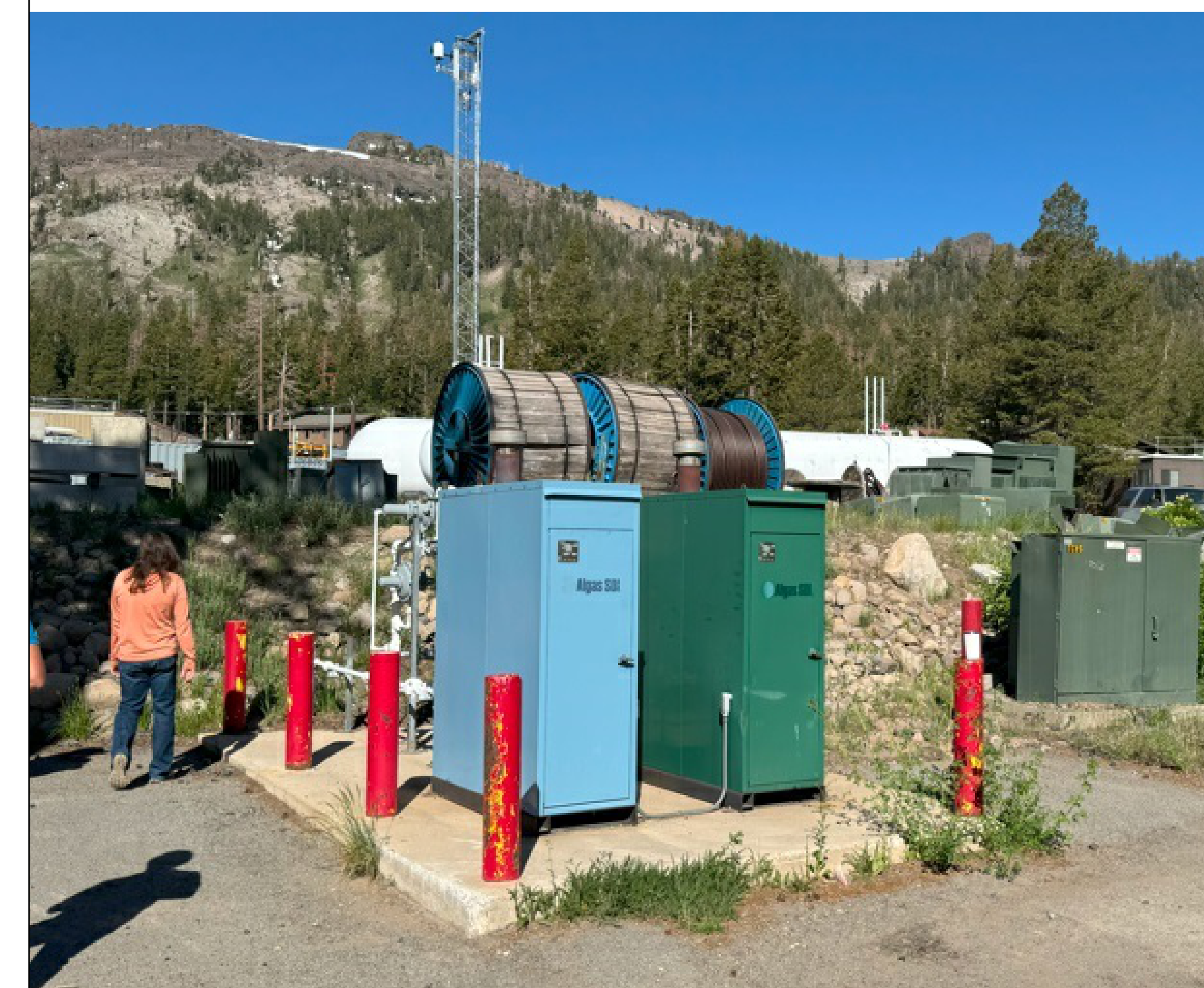
SITE: LOOKING NORTHWEST
