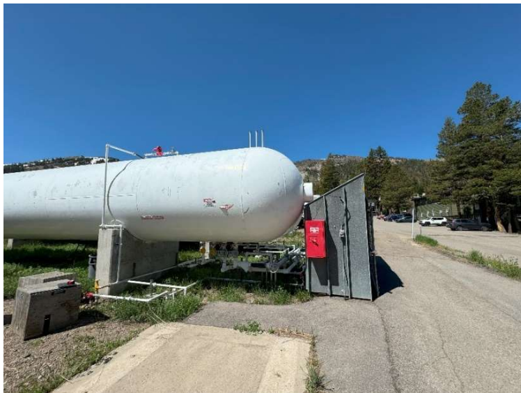
Figure 3.3: Existing Storage Tanks (looking west)
