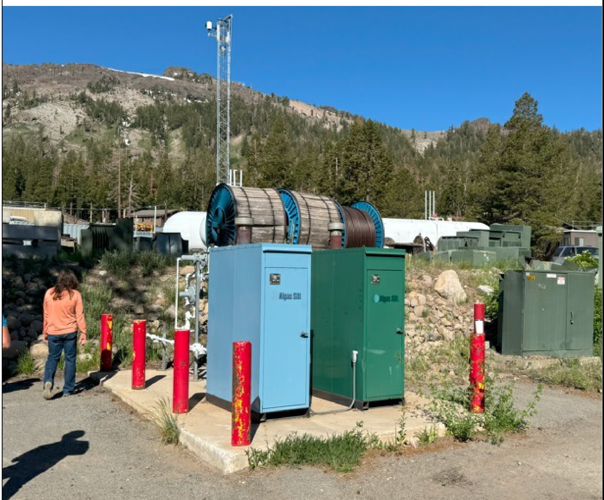
SITE: LOOKING NORTHWEST
