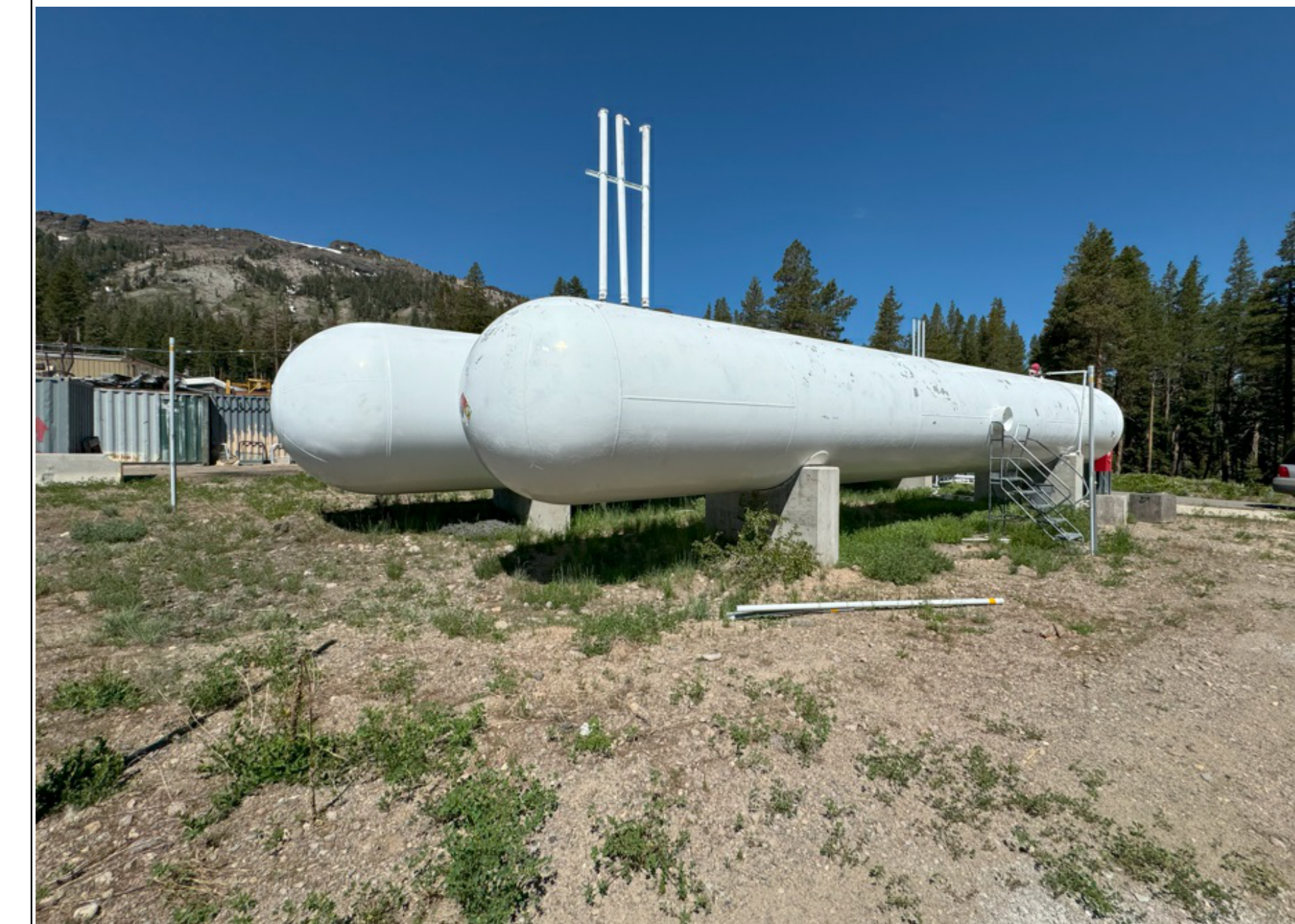
SITE: LOOKING NORTHWEST
